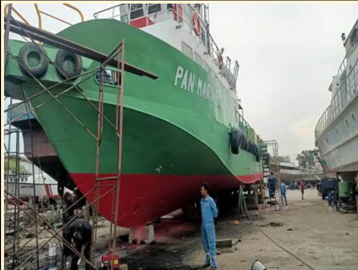
Full coat Interspeed (BQA377) red at underwater area.
