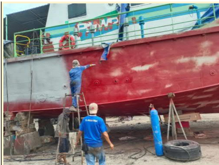
Application Touch up coat Intergard 263 (FAJ0034/A262) Light grey at Topside area.
