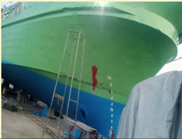
Full coat Interspeed 376 (BQA372) Blue at underwater area.
