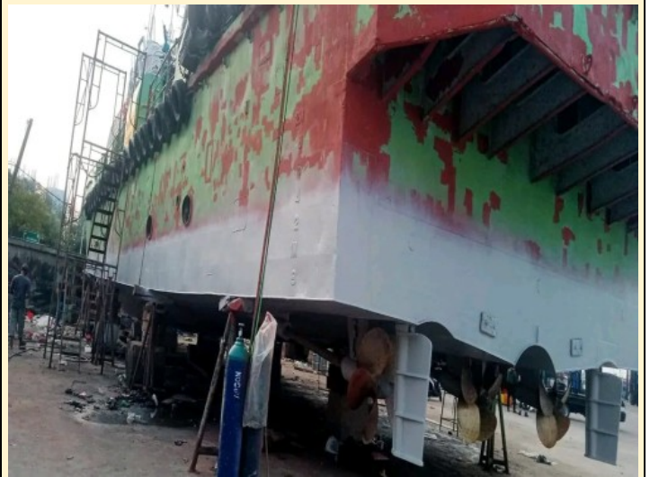
Full coat Intergard 263 (FAJ034/A) Light grey at underwater area
