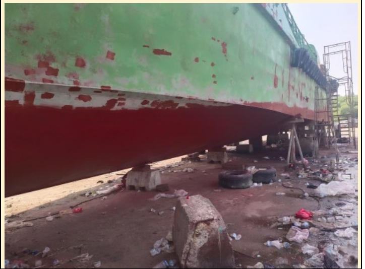
Full coat Intertuf 262 (KHA303/A) Red at underwater area
