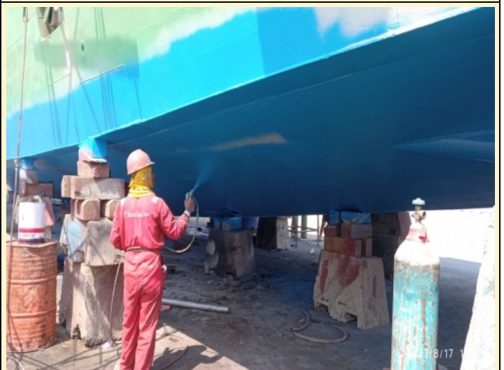
Painting 3rd coat Interspeed 376 Blue (BQA372) in underwater area.
