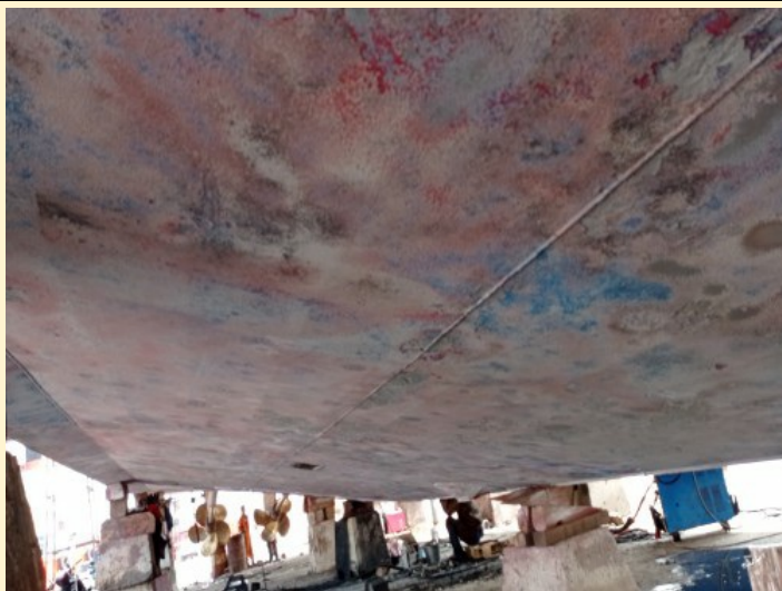
Showing result sweepblast on underwater area.
