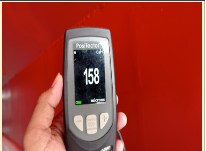
Check DFT on the first layer of Intertuf 262 Red
