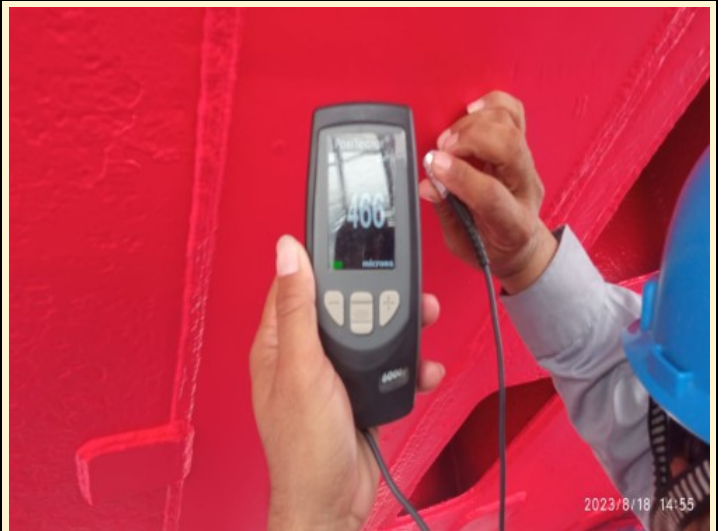
Check DFT on the finish layer Interspeed 376 Red.
