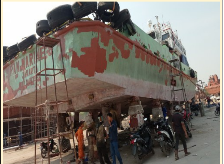
Showing result sweepblast on underwater area.
