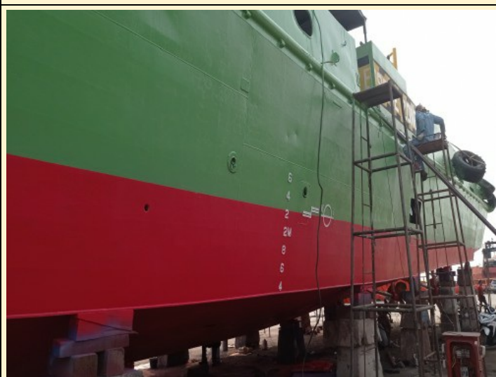
Final condition of Pan Marine 8
