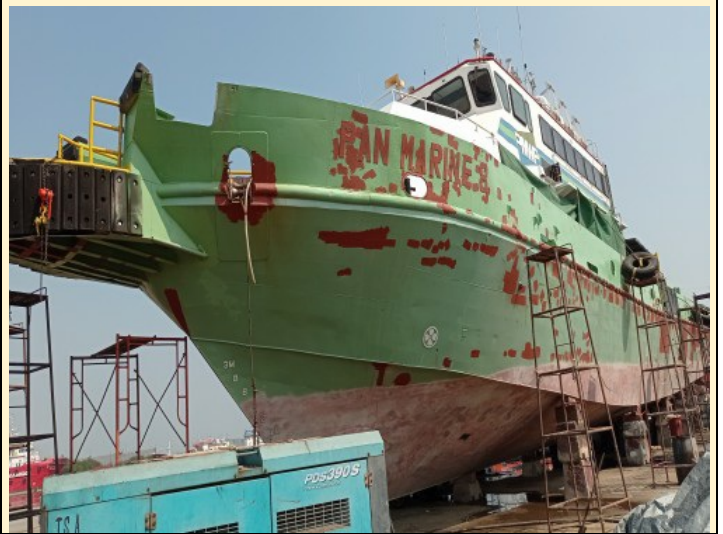
Showing result sweepblast on underwater area.
